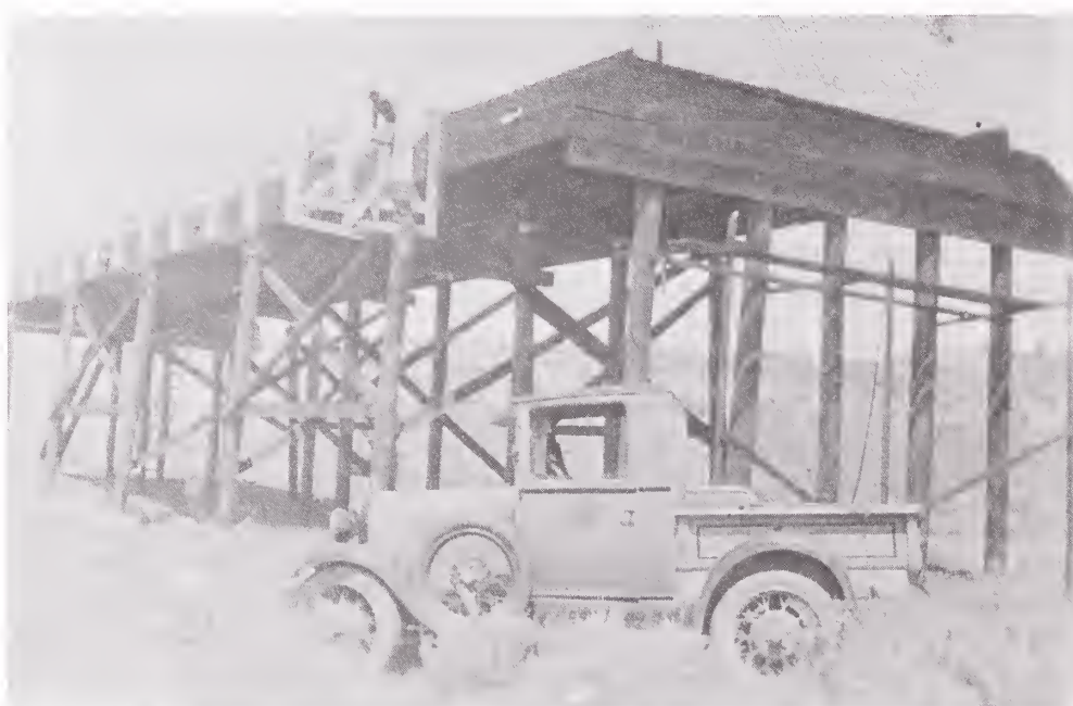
A standard timber bridge during construction in 1929. The bridge was located in the vicinity of Miles City and was built by Frank Robbins for the Montana Highway Commission (photograph courtesy of Bob Robbins).
